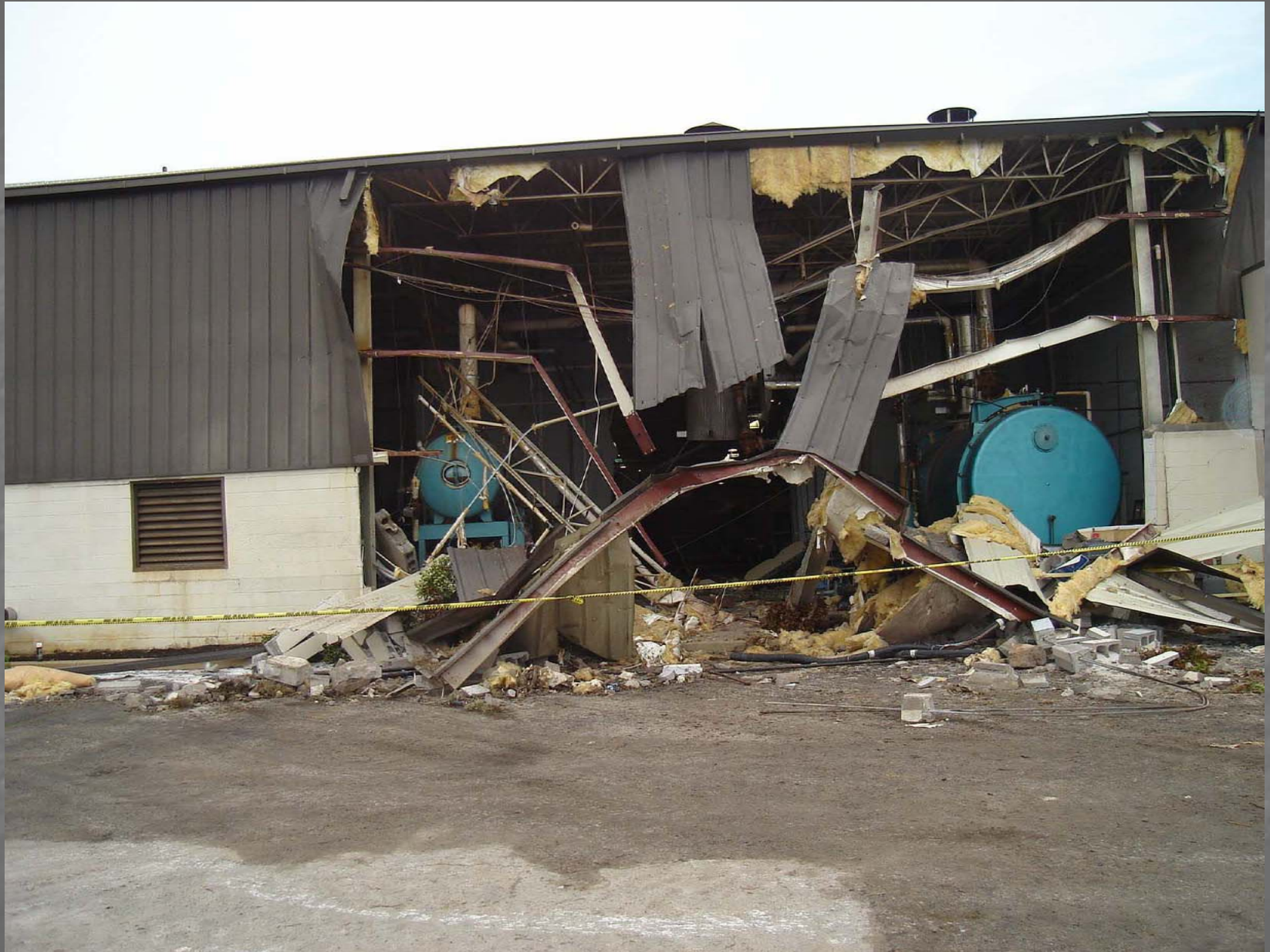
View of East Wall from Outside Plant
