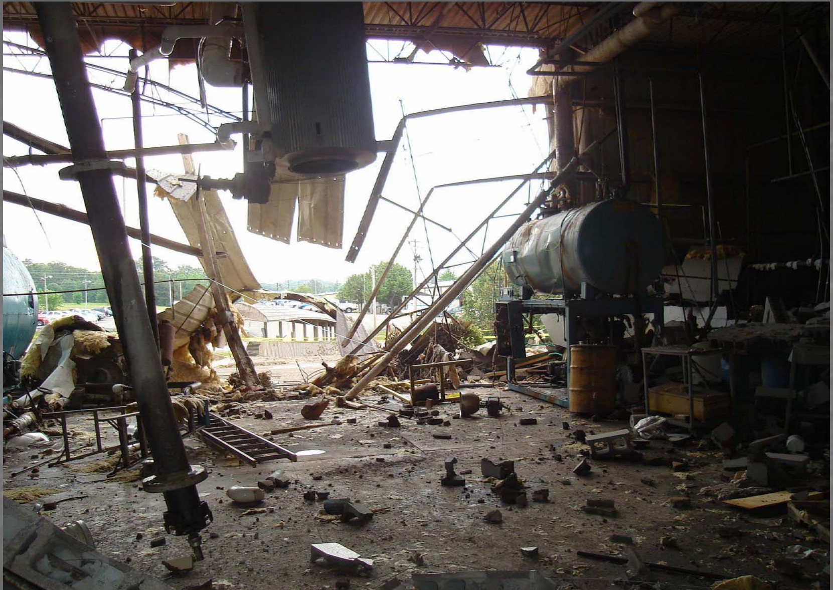
Knocked Down Exterior Wall Viewed from Inside Boiler Room (East Wall)
