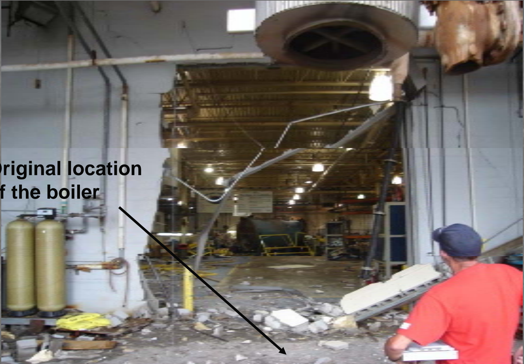
Hole Created by Boiler through Roll Up Door Wall (West Wall)
